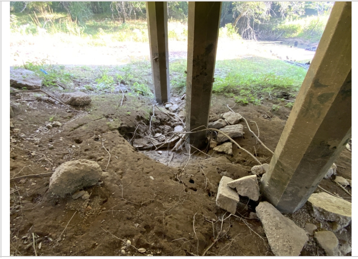
Scour hole around pile 2 Bt 2, 3ft deep, 5ft diameter
