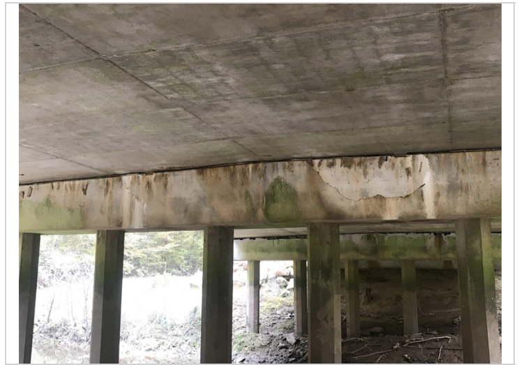
Delam, bent 3, back face.
