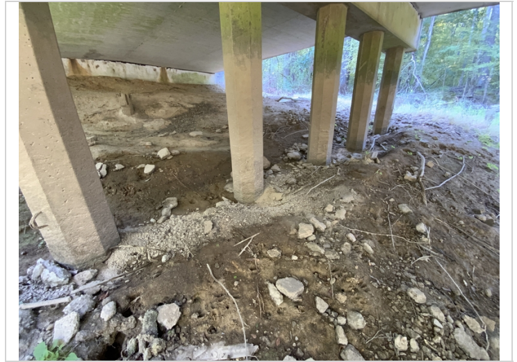
Bent 4, minor erosion around all piles. 1ft deep
