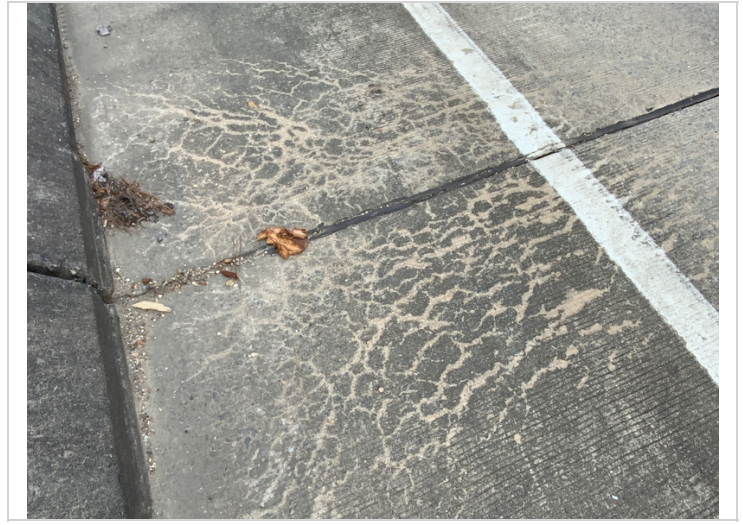
All corners of slabs over bents have map cracking.
