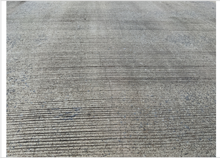
Span 1 longitudinal cracks up to 0.020". Common all spans.
