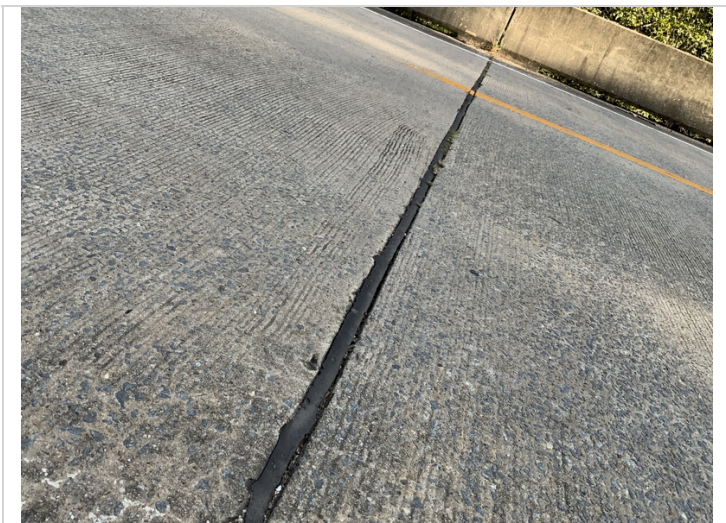
Bent 3 joint seal loss of bond.
